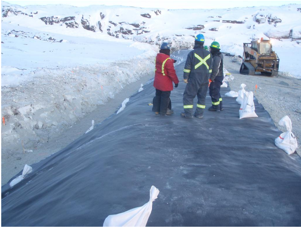
Photo 8: Layfield gathering atop the geotextile under liner
