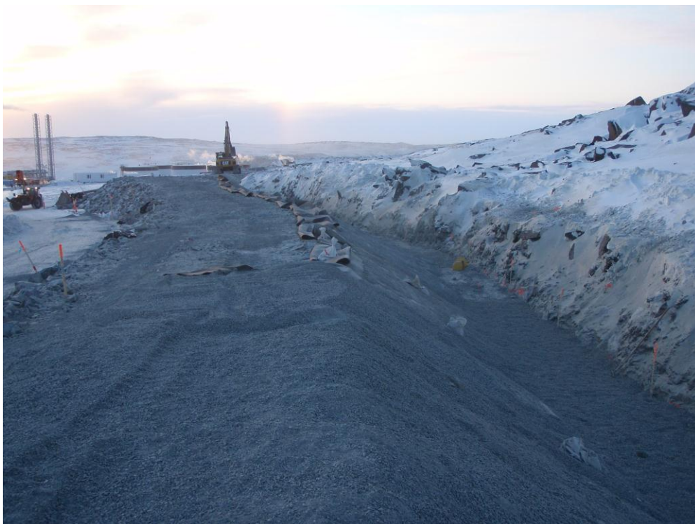
Photo 7: Crush placed atop the lower geotextile at the Doris North Diversion Berm
